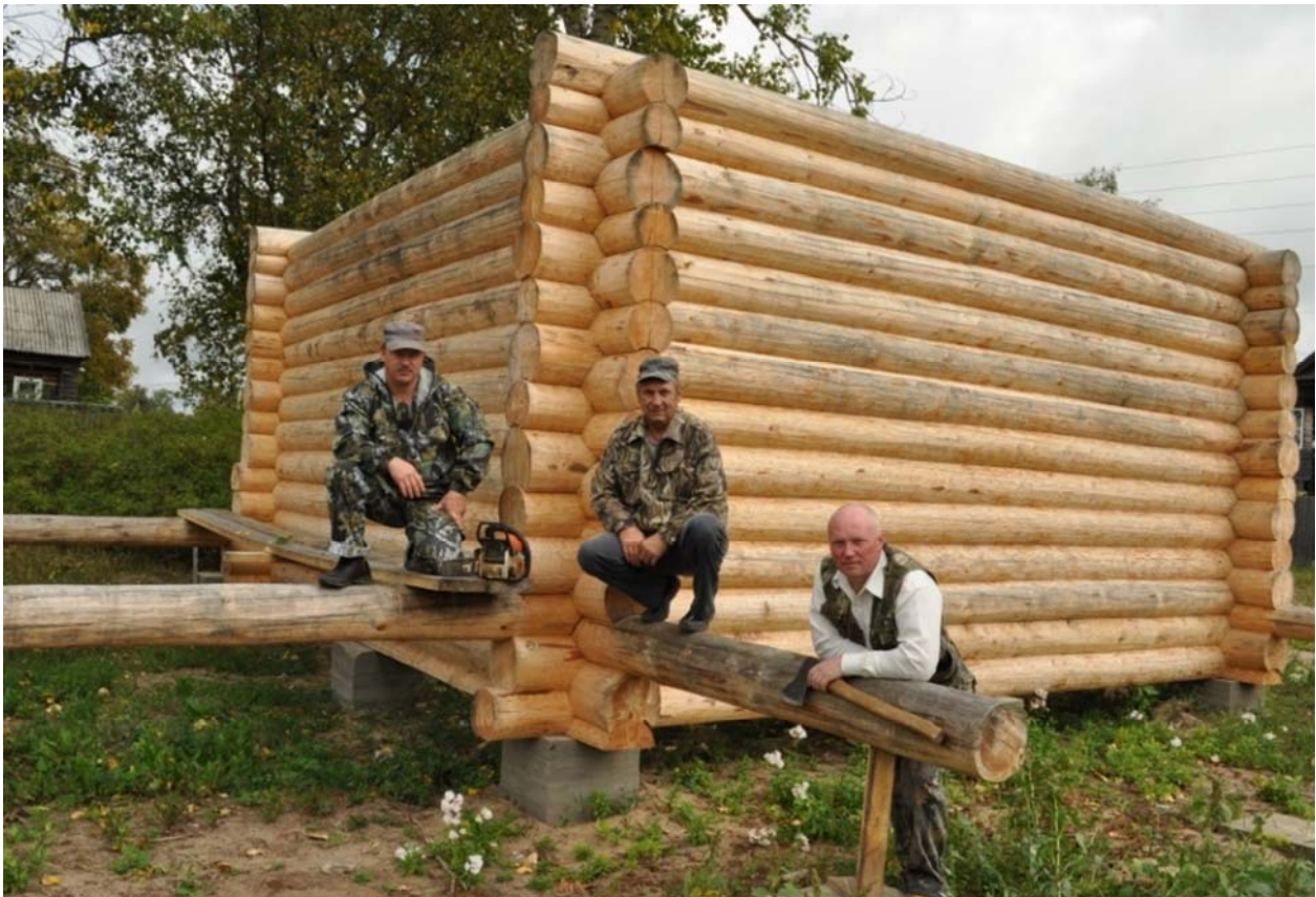
Photo 5. Kologriv, Kostroma Region, bank of the Unzha River. Otkhodnik carpenters, who pre-fabricate log cabin kits at home, deliver them to the customer in the suburbs of major cities, and erect houses from them. The high quality of their work can be seen even in the picture: the logs fit so tightly together that there is not a single gap between them. Every log is placed in the cribwork with due consideration for the growth characteristics of the tree and potential future checking (the splits will appear on the downside or inside surface of the logs). The photo shows the central cribwork of the future house; the beams on which the builders are sitting are the bottom (floor) connection of the cribwork with the exterior walls of the big 10x10 m house. The top beams and the roof rafters are not yet in place. Photo by Juri Plusnin, August 2014.
