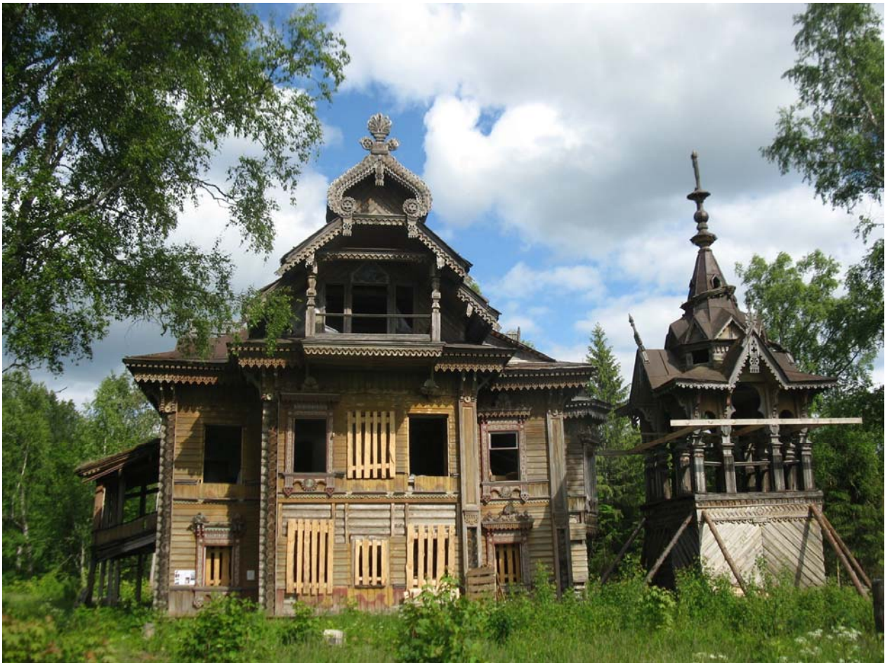
Photo 3. An old residential house (actually a wooden palace) built in the village of Astashevo in Chukhloma district of the Kostroma Province. A local peasant otkhodnik and cabinet-maker constructed the building at the end of the 19 th century. He made a fortune as leader of Chukhloma carpenter teams ( artels ) that worked in the capitals. The house has long been abandoned. The tower in the forefront has been dismantled from the roof to be reconstructed. Currently, local and metropolitan volunteers are restoring the building. Photo by Natalia Zhidkevich, June 2011.
