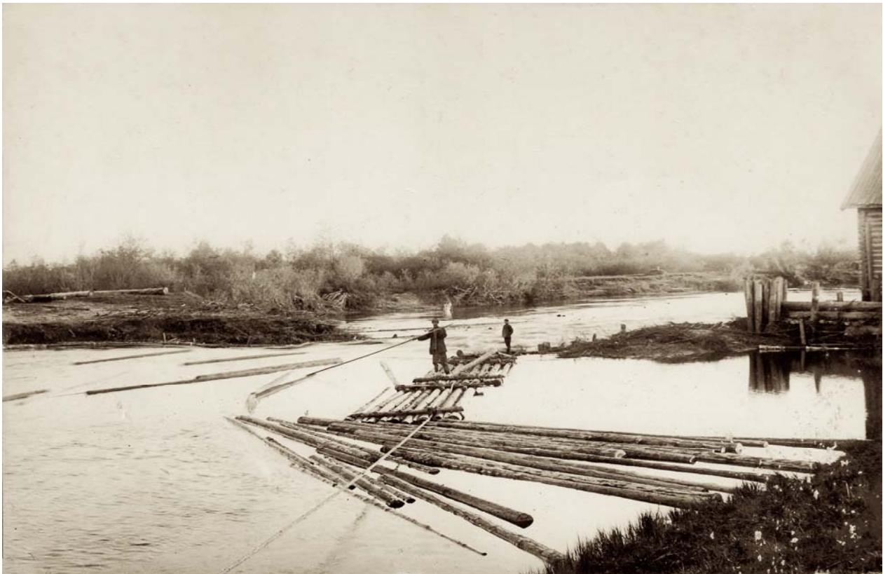
Photo 2. Raftsmen on the Vetluga River in the Kostroma Province; first half of the 19 th century. The picture made by Zinoviy Vinogradov, a photographer from Nizhny Novgorod, shows Vetluga raftsmen at work collecting logs from a smashed raft and tying a new raft right on the water (the remains of the raft are roped to the bank of the backwater where there is no current). They had to do this kind of work often because the swift spring current of the winding Vetluga smashed the rafts against the riverbanks and islands. Photo courtesy of Prof. N.V. Morokhin (Nizhny Novgorod).
