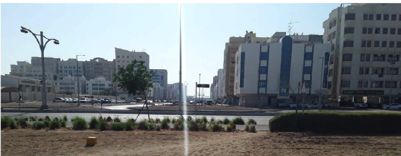
Figure 2: A picture of Al-Anwar main road and the other residential buildings.
