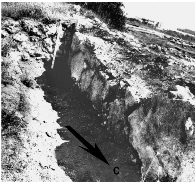
Figure 5: Western fortress wall. Exterior façade. View from the west.
