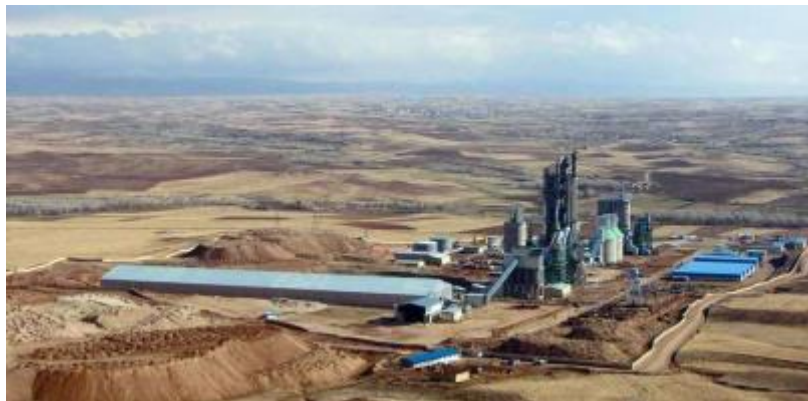
Figure 9. Shahrak iron ore concentrate Plant
