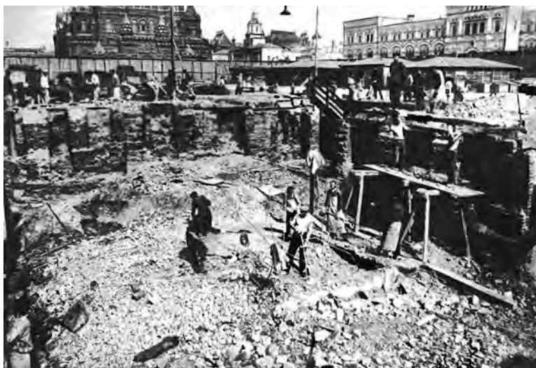
FIGURE 11. Foundation pit for the permanent mausoleum, 1929, in Kotyrev, Mavzolei , 137.
