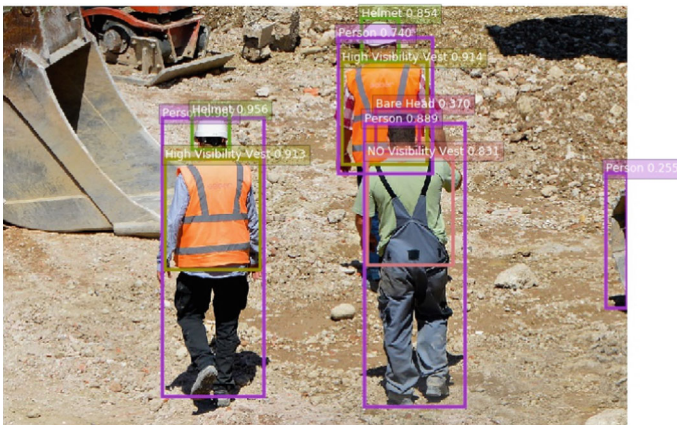
Fig. 8 Real-time field monitoring and PPE detection on workers
